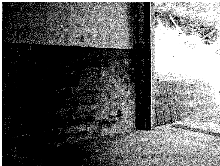
Hornby Is Fire Hall – soil to be removed from contact with wall and exterior buttresses to be constructed on exterior side.
